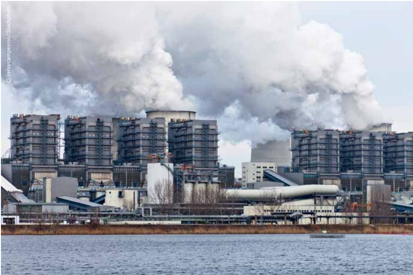
FIGURE 2: Coal-fired electricity-generating stations are the world's largest point sources of both CO 2 and SO 2 . Jänschwalde, near Peitz in Brandenburg (very close to the Polish border), is Germany's largest lignite-fueled station with three gigawatts of installed electrical capacity; it generates annually 22 terawatt-hours of electricity and it was to be the site of a large-scale carbon capture and sequestration project that was cancelled in 2011.
